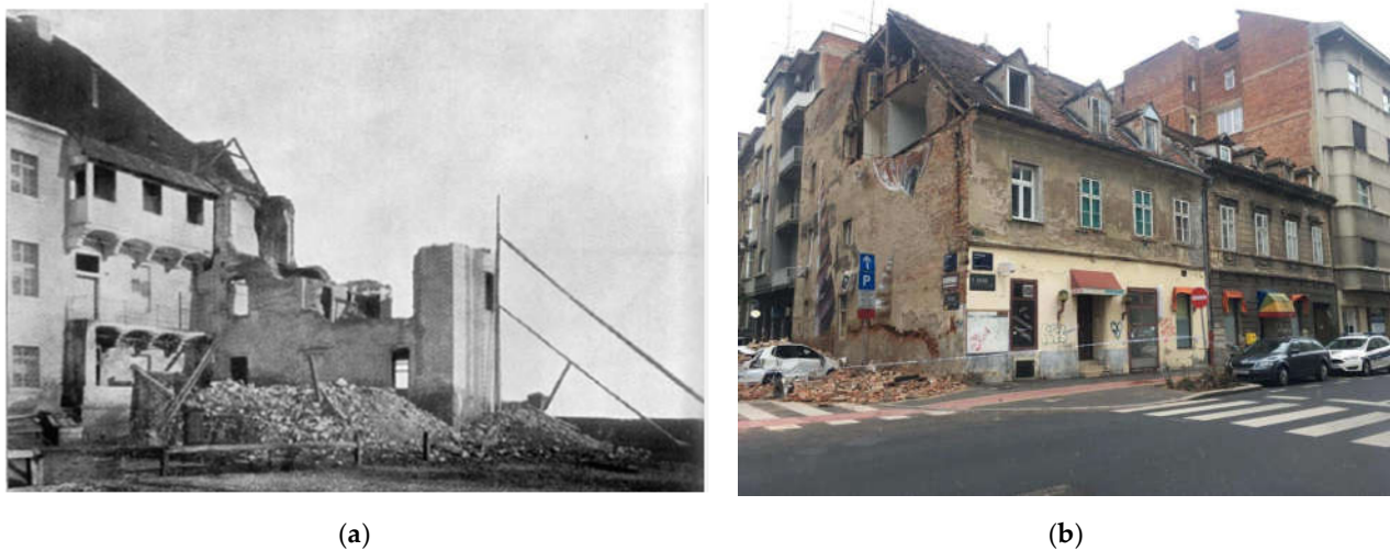
Figure 1. Building devastation after: (a) 1880 Zagreb earthquake [4] Reproduced with permission from Zagreb City Museum, 2022.; (b) 2020 Zagreb earthquake (author's figures).
