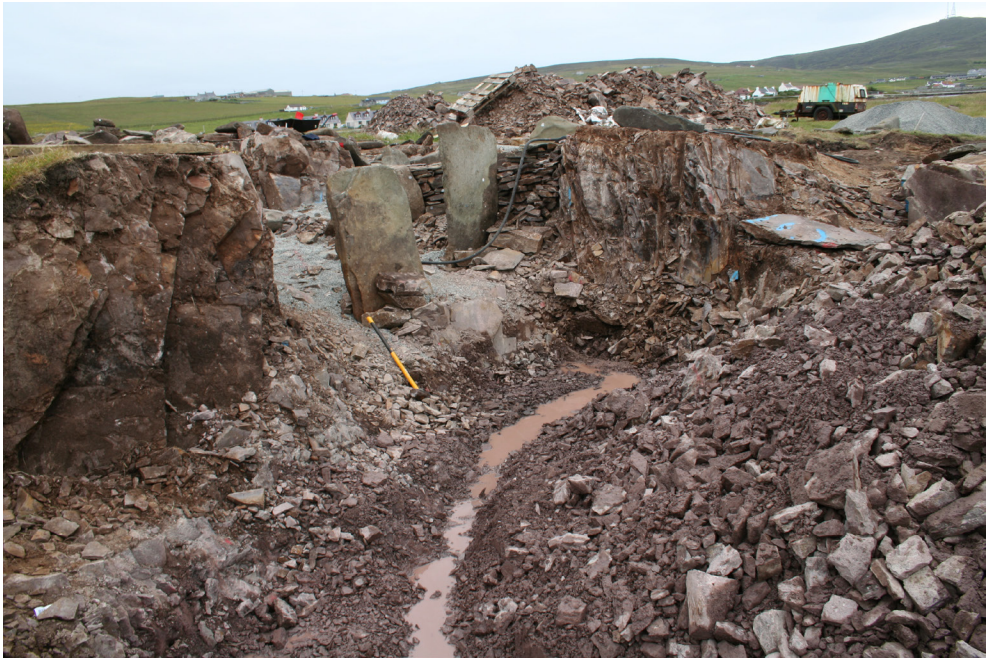
Figure 12: The reconstruction site during the project.
