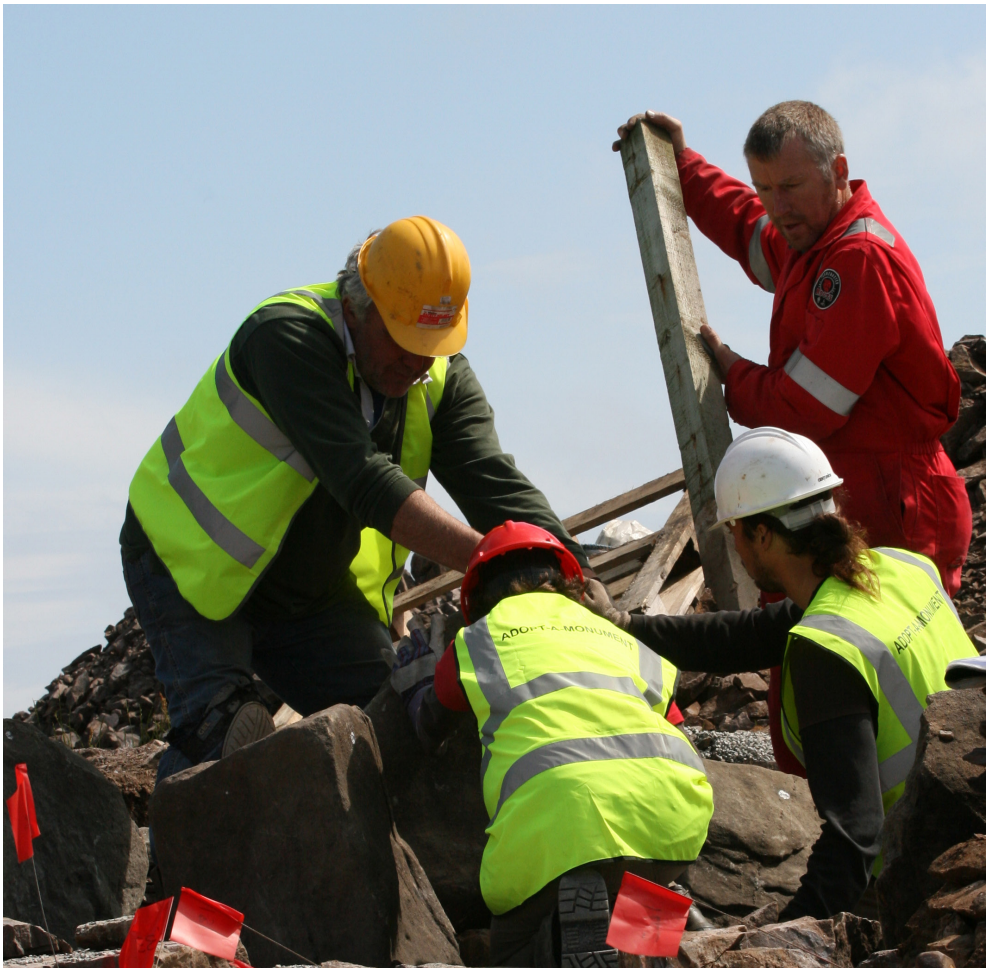
Figure 11: Volunteers work with contractors to place the orthostats in position.
