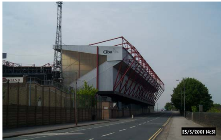
Figure 2: Side elevation of the Midland Road Stand
