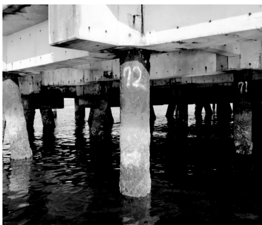
Fig. 8 A group of pipe piles supporting a wharf
