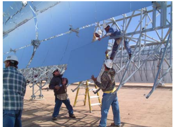
Assembly of the reflector panels
