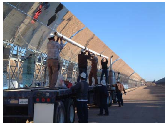
Assembly of the absorber tube
