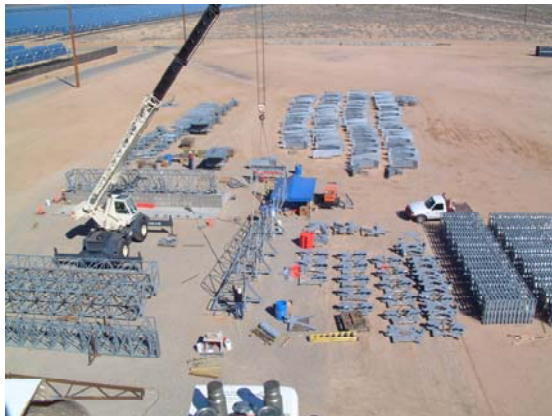
Construction site at the power plant compound in the USA
