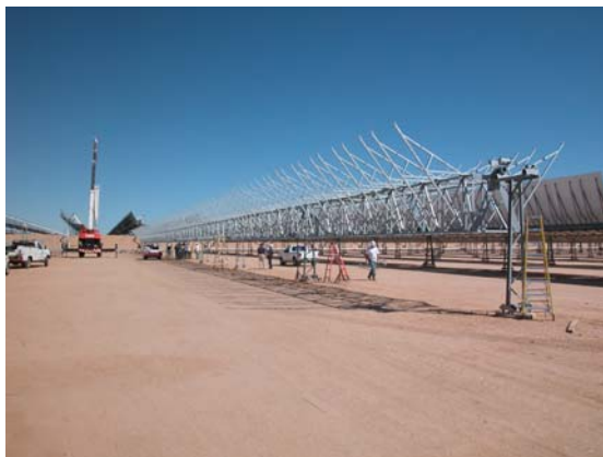
Assembly of the field framework and reflectors
