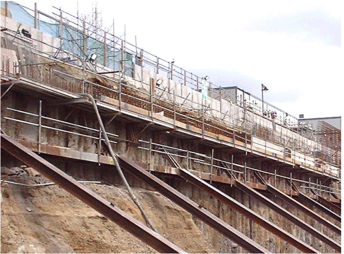
PLATE 3.7 Berm with raking props at Canary Wharf, London
