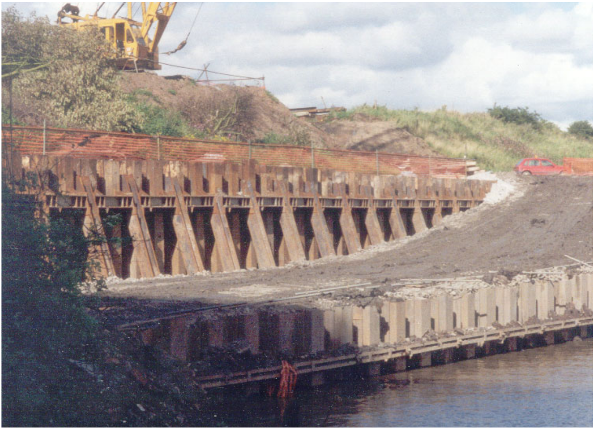
PLATE 3.5 Various support systems to sheet pile walls at Thelwall Viaduct, Merseyside
