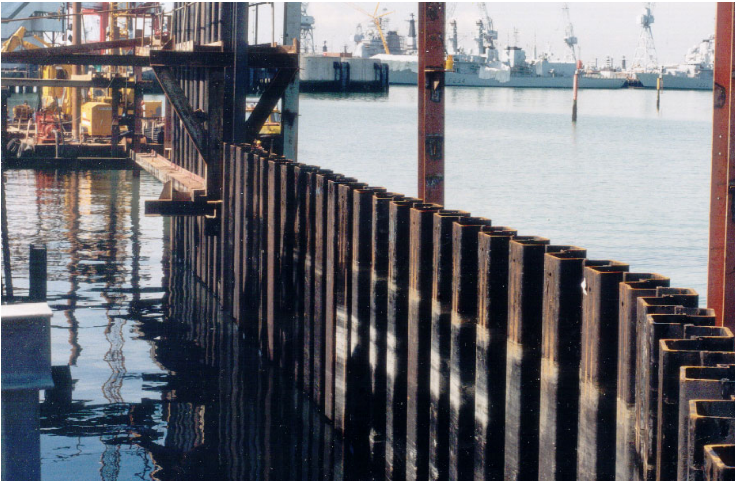
PLATE C.1 Sheet pile wall installation, Portsmouth Harbour (courtesy of Corus)
