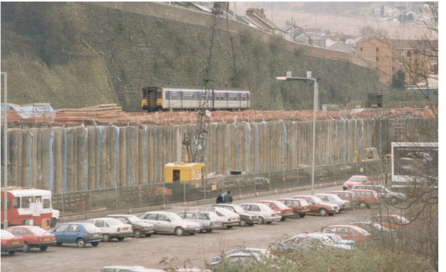
PLATE C.2 Contiguous bored piled wall (courtesy of Bachy Soletanche Limited)
