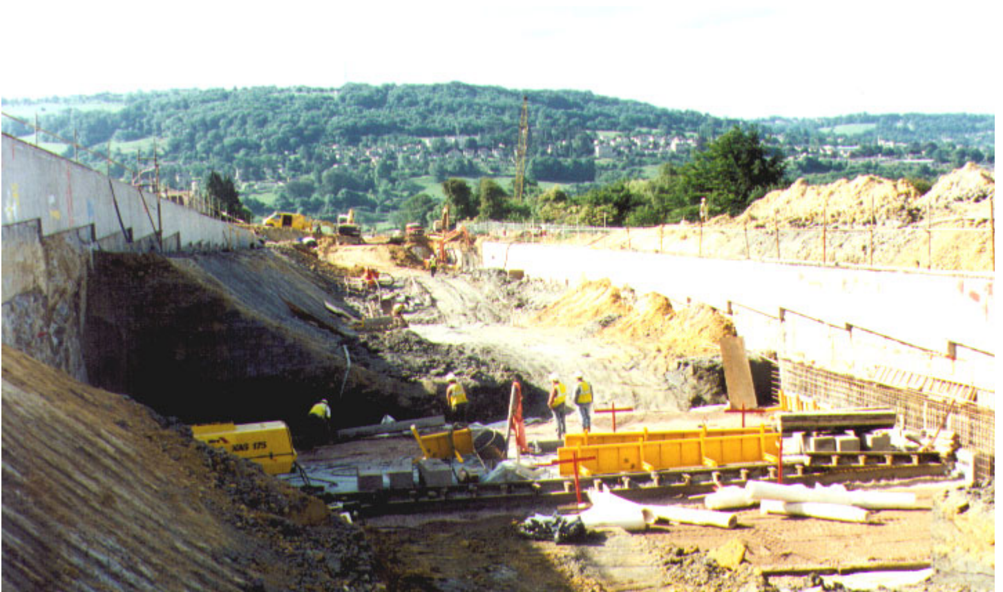
PLATE 3.8 Berm with low level permanent propping at Batheaston Bypass
