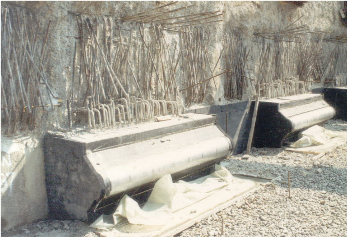
PLATE 3.11 Hinged joint: A406 North Circular Road, London
