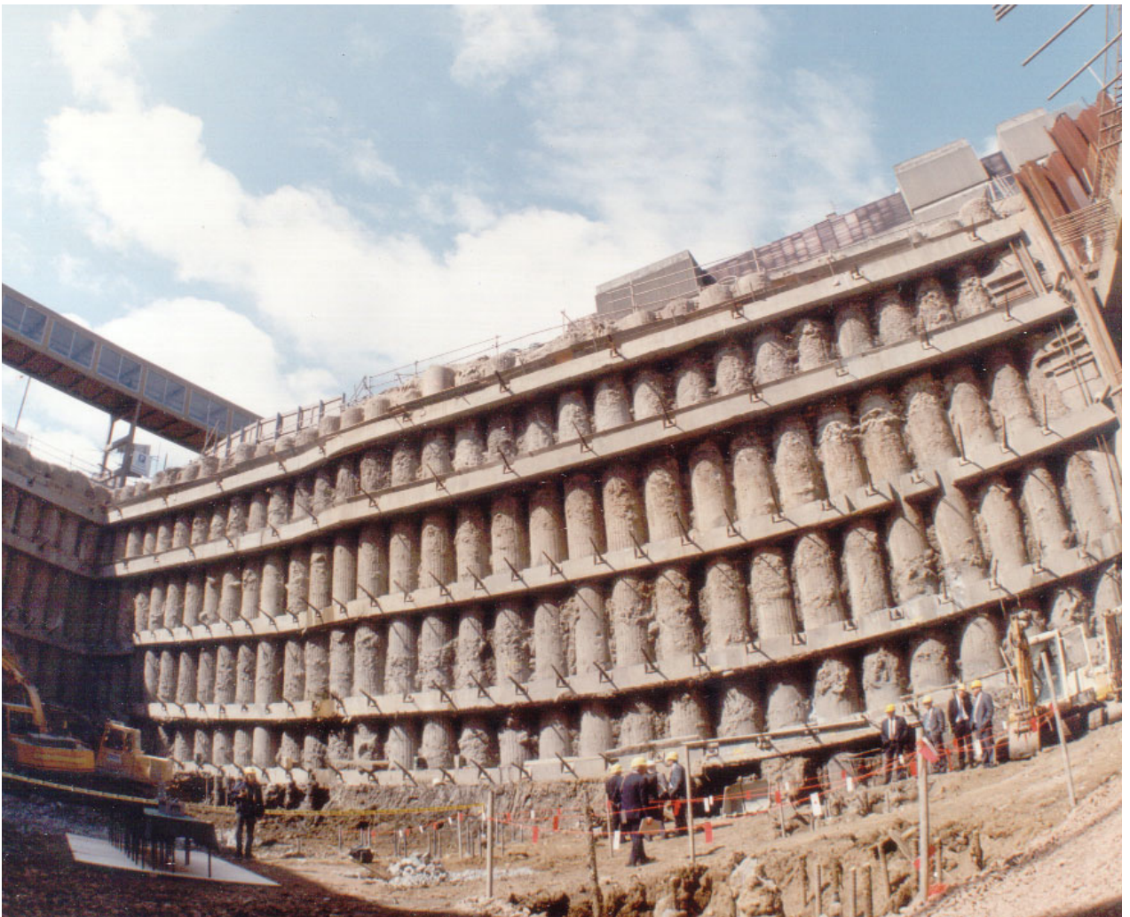
PLATE 3.9 Anchored contiguous bored pile wall
