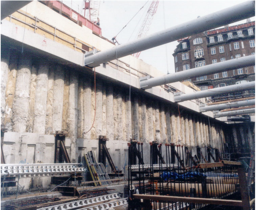
PLATE 3.3 Bottom up construction sequence
