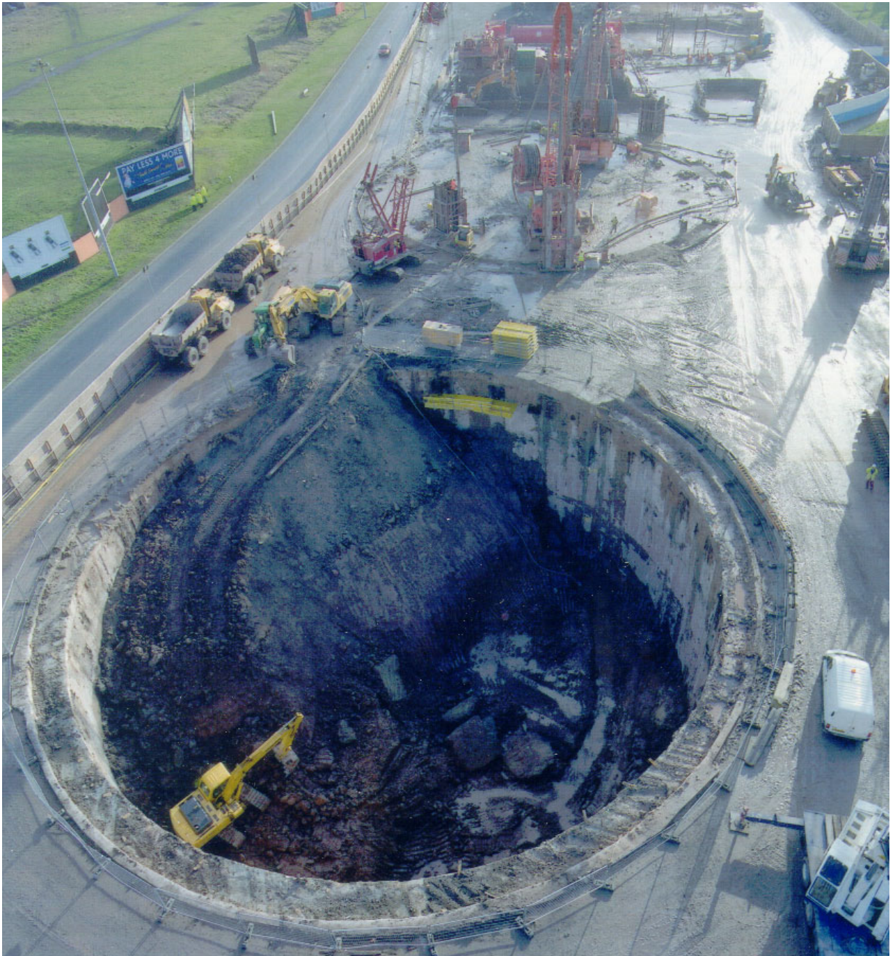
PLATE 3.4 Circular shaft under construction at Blackpool, Lancashire
