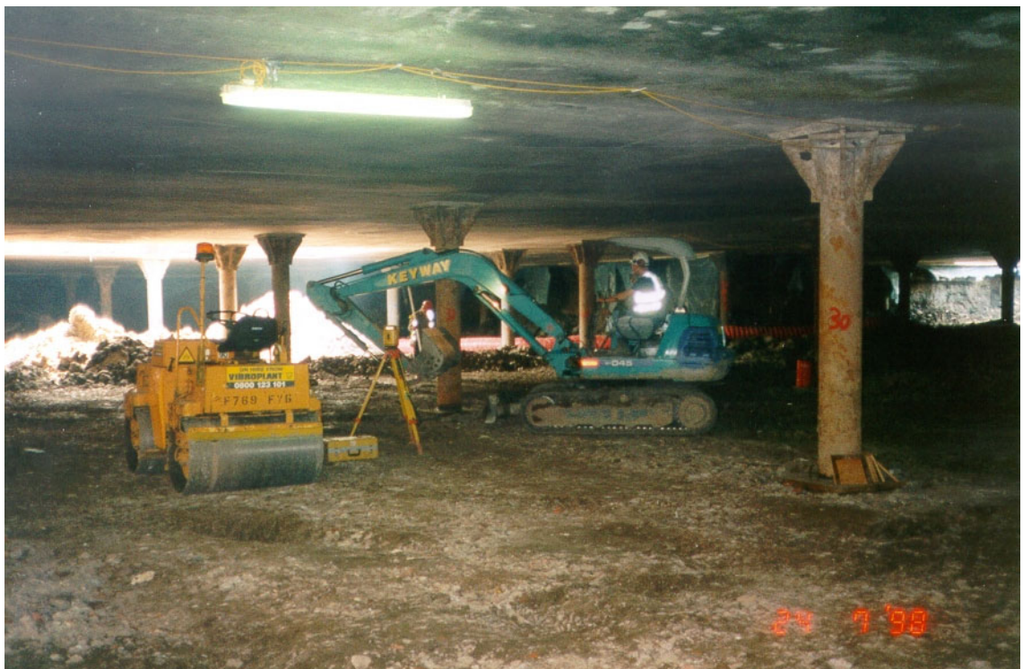
PLATE 3.2 Top down construction sequence.
