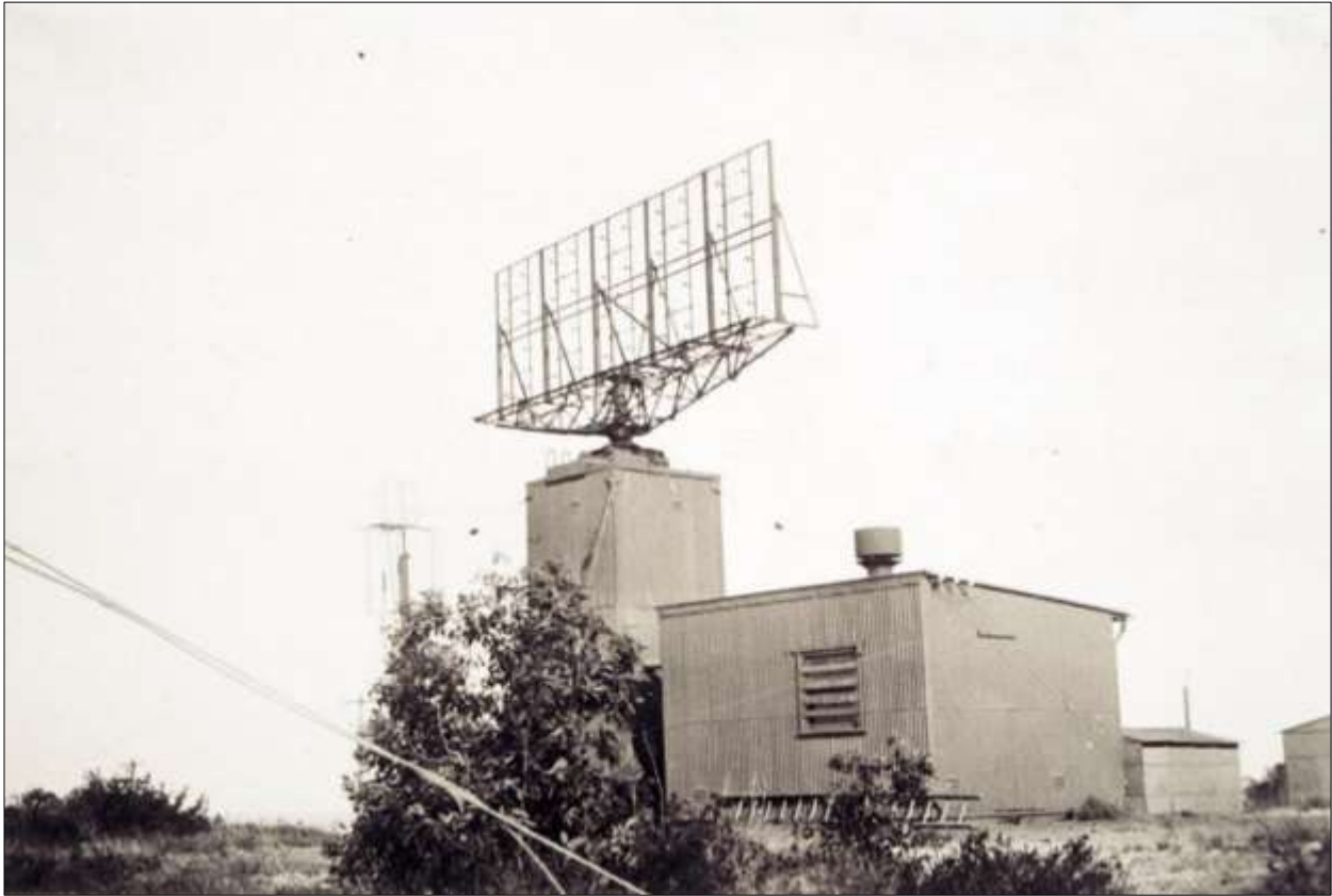
Figure 1: The 200 MHz COL Mk.V radar at Collaroy Plateau in early 1946. The view is looking toward the east with the control room in the foreground. The COL radar was a British design with the tower structure built by the NSW Government Railways (after Dellit, 2000: 48).
