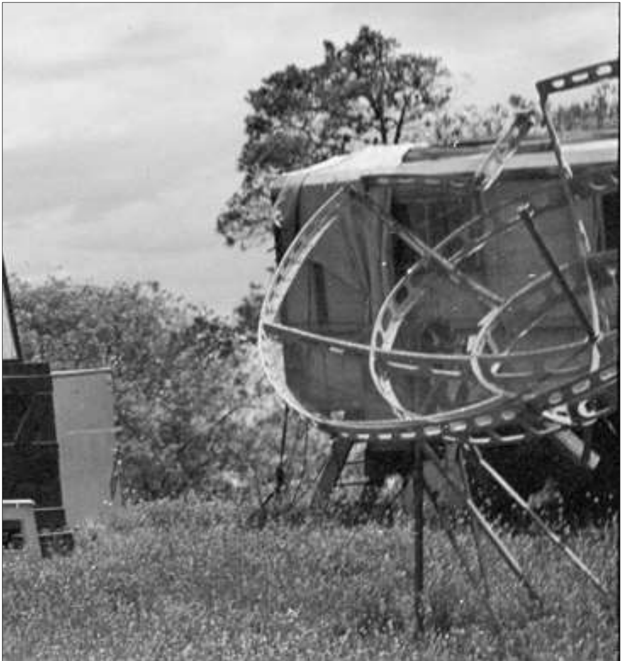
Figure 12: One of the AN/TPS-3 aerials at Potts Hill in November 1951 showing damage to one of the aluminium segments (adapted from RAIA, B2639).
