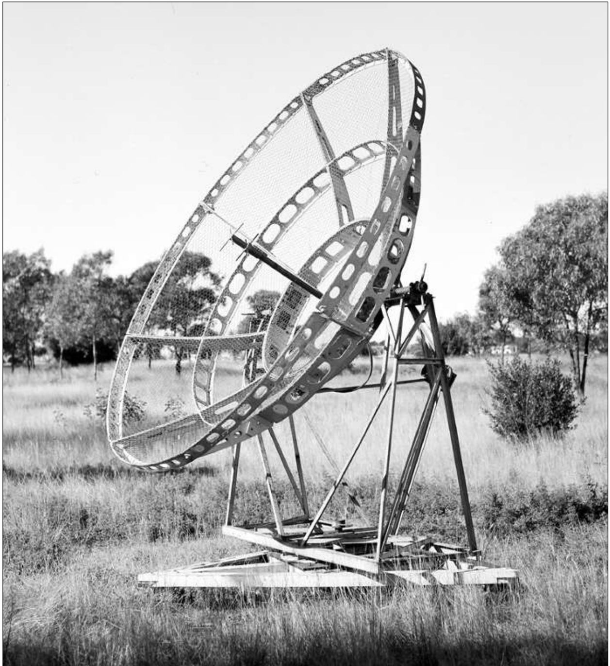
Figure 8: An AN/TPS-3 Aerial at Potts Hill field station in 1949. The horizontal and vertically polarised dipoles at the prime focus are visible (courtesy: RAIA, B1511).
