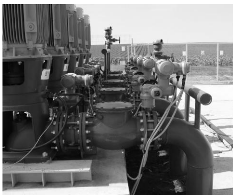
Figure 5 The rehabilitated hydraulic installation of the pumping station SPP1b
