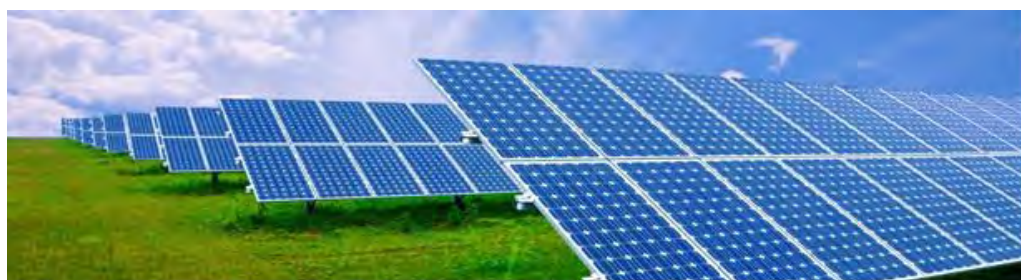
Fig. 1. Solar power plant.
