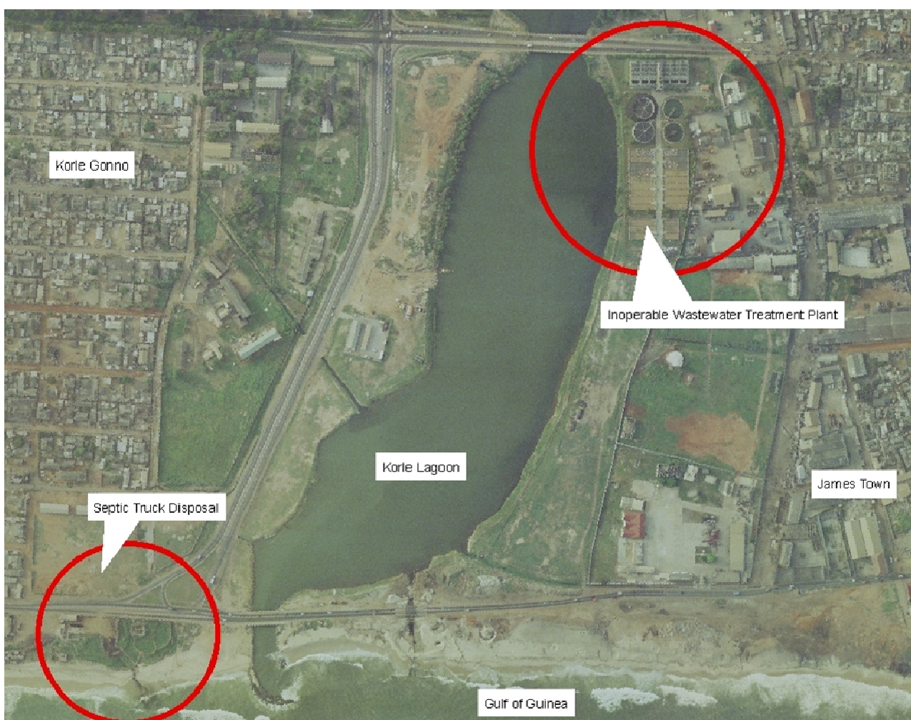
Figure 3.7 Inoperable Wastewater Treatment and Septic Truck Disposal
