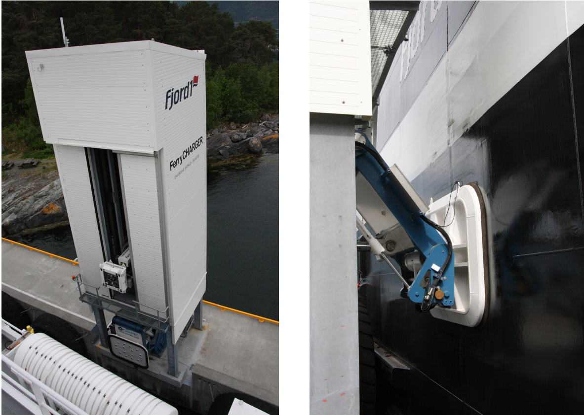
Figure 21: The charging tower "FerryCharger" and automated docking solution at the Anda-Lote site. Source: Teknisk Ukeblad
