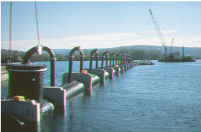
Figure 2: Diffuser configuration example (here floating before installation on the bottom). The risers are bended sideward and the ports are still closed.
