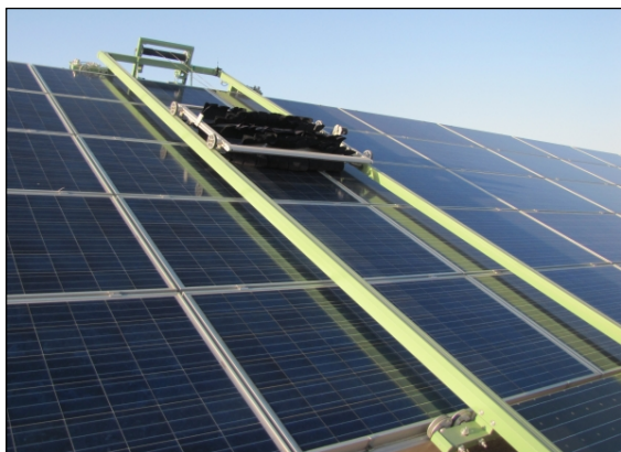
Figure 10: Mitigation as dust cleaning solution in an automated brush-cleaning system in Israel [9]
