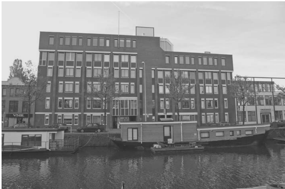
Figure 1. The existing façade was kept
