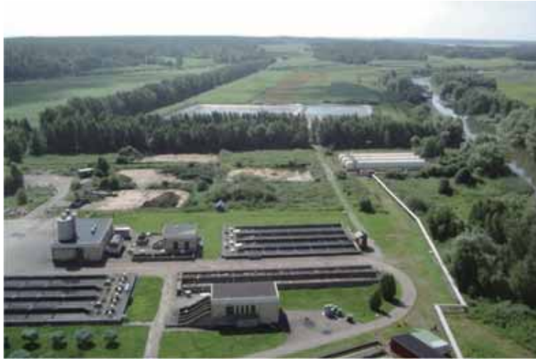
Fig. 9.1 A 75 ha willow phytoremediation system at Enköping, Sweden. Foreground: wastewater treatment plant; middle: ponds for winter storage of wastewater; background: willow fields irrigated by wastewater from sludge.
