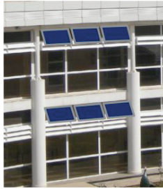
Fig. 3. One of the integration scenarios: Substituting the overhangs by BIPV.
