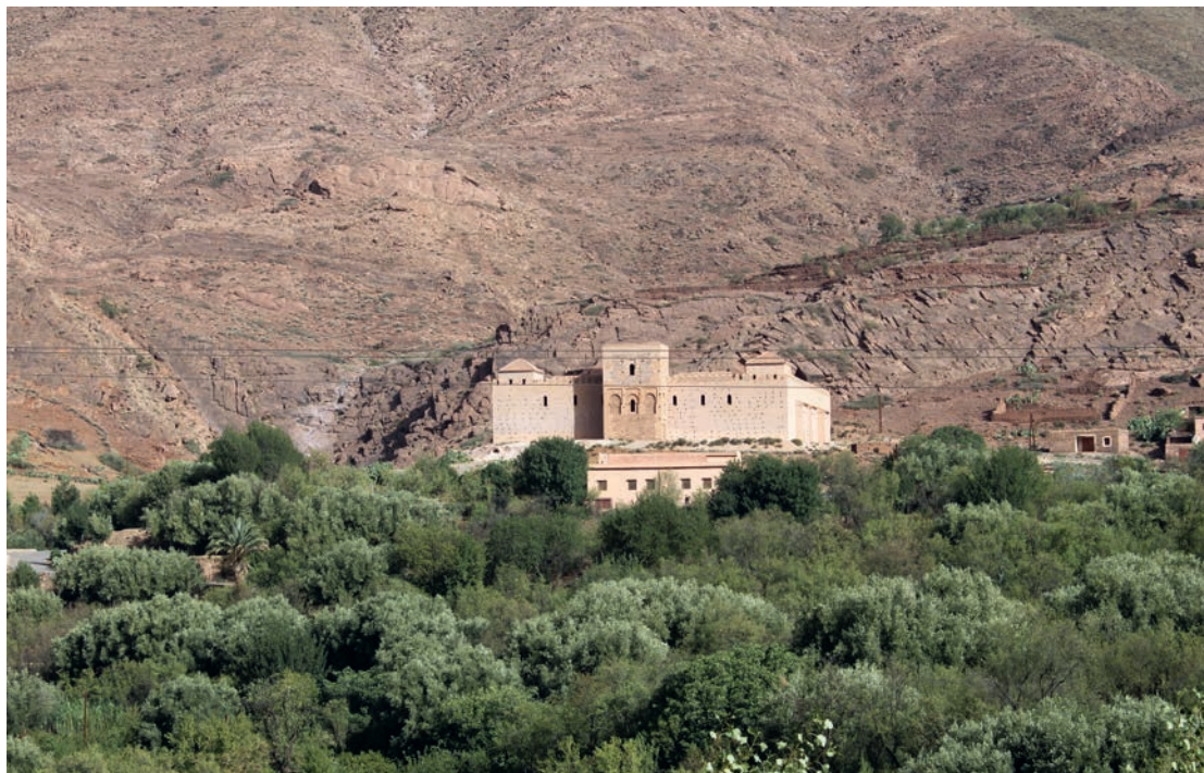
Fig. 1: Mosque of Tinmal. General view from the south
