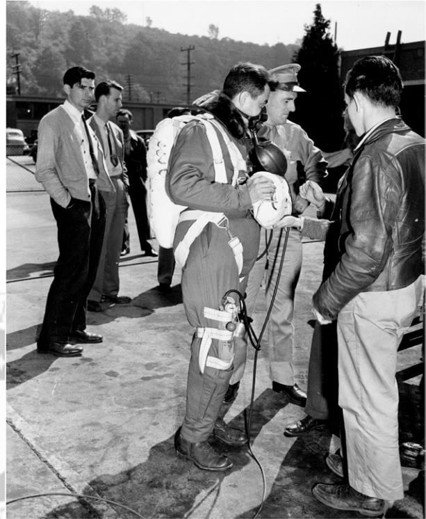
Fig. 1. Lt. Col. Lovelace wears a rebreathing pressure mask, type H-2 oxygen bottles, and type T-5 parachute before his high-altitude jump on June 24, 1943. Association by Ingenta
