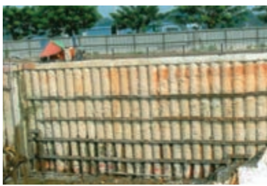
SGE Jacked Anchors for 10-12m CBP Retaining Wall, SMART Tunnel
