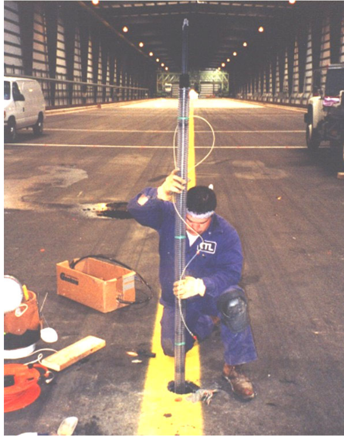
FIGURE 15 Snap MDD Installation.
