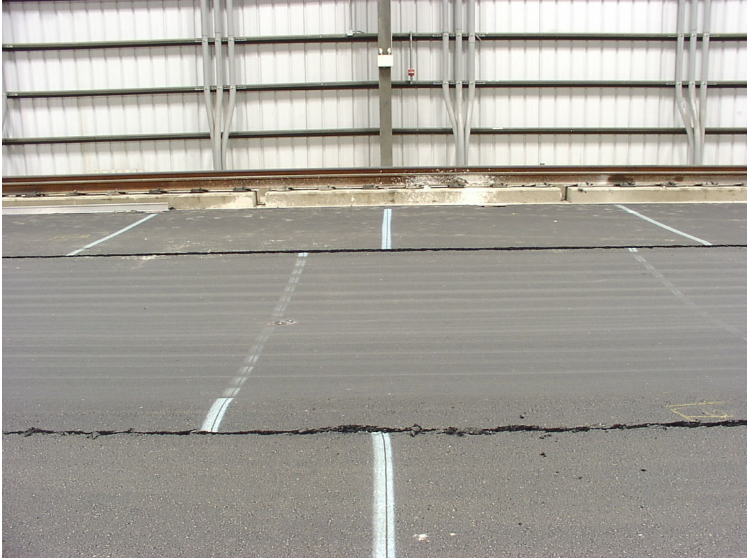
FIGURE 8 Pavement Displacement.
