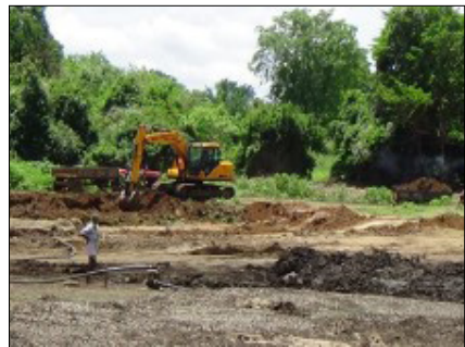
Removal of silt Kaporiggama STC Photo credit: IUCN
