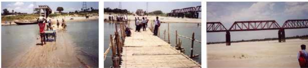
a. Gorai River passing b. Gorai east bank c. Gorai Railway Bridge Figure 6. Changing pattern of Gorai River morphology in 2003 (a, b, c)
