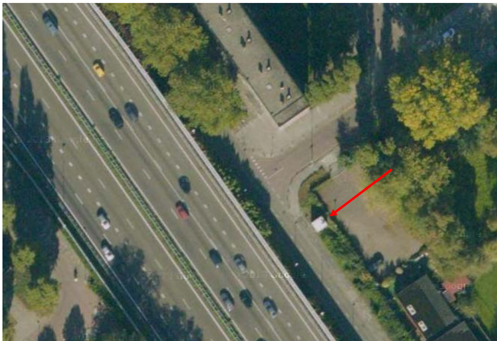
Figure A.4: A13 Motorway and location of the monitoring site.
