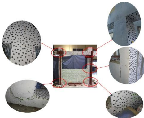
Fig. 3 Damages to RC partial infill frame subjected to slow-cyclic loading (Kaushik et al. 2018)
