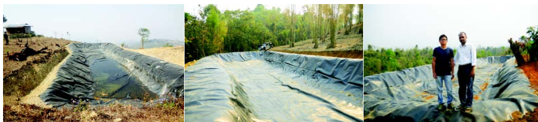
Water harvesting structure constructed at Longleng, Peren and Dimapur
