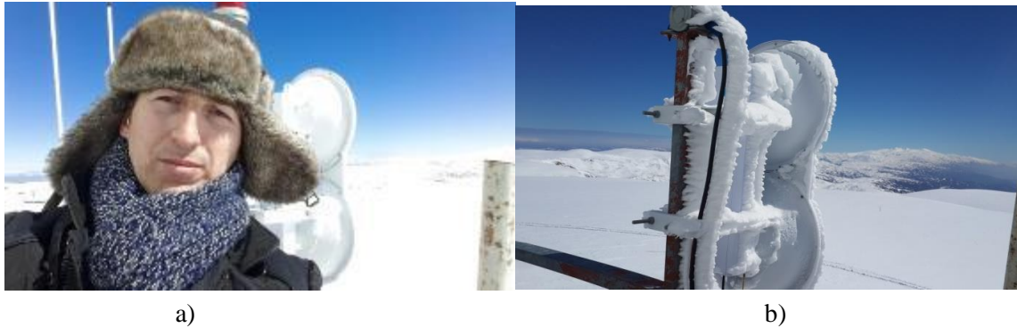
Figure 9. ErzincanRefahiyeVabel VOR Station AirFiber 5 setup phase
