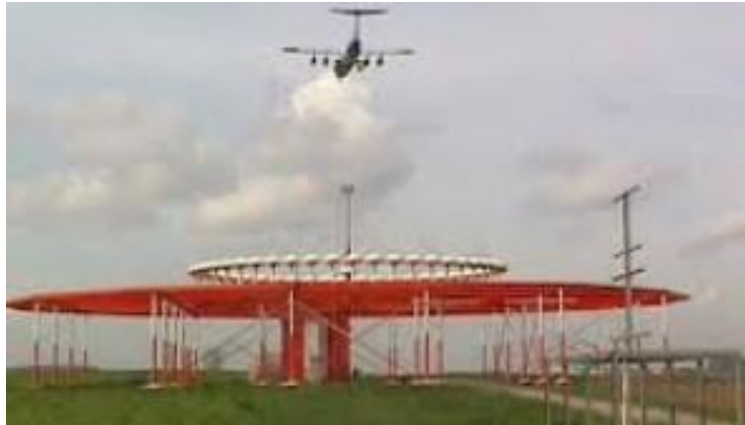
Figure 1. Outside view of station VOR (HAVALİMAN, 2016).
