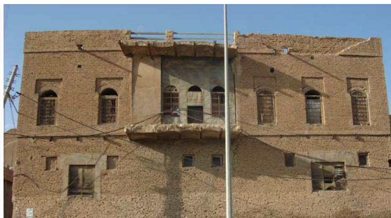
Figure 6.10: Using Brick as Basic Building Material in the Traditional Period (before 1930) Source: The Author
