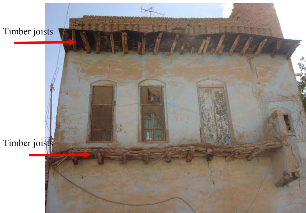
Figure 6.11: Traditional Roofing Materials Based on Timber Joists Covered by Matting Source: The Author
