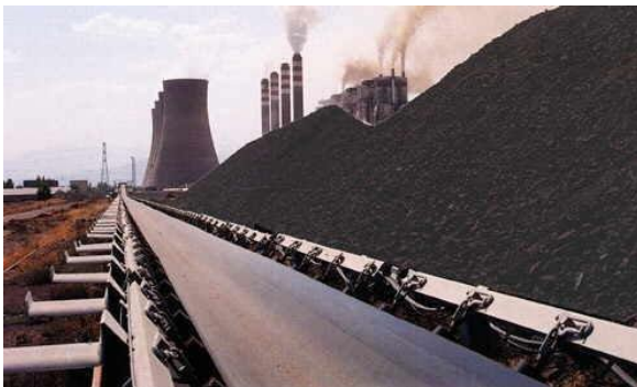
Figure 1. A typical belt conveyor used for transport (ÖZERBAND, 2015)
