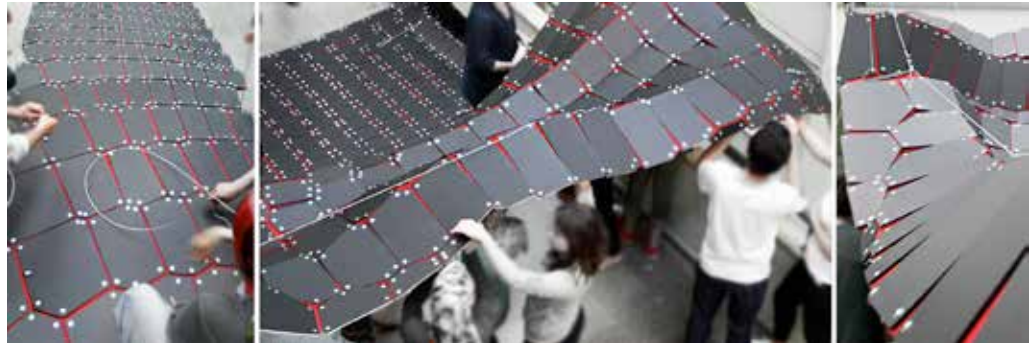
Figure 15 Re_Flex Patterning; Third and final day, installation.
