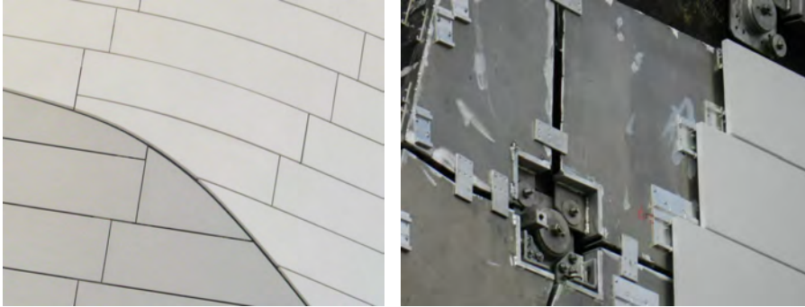
Figure 1.3: Complex and curved façade cladding used in the new building for Fondation Louis Vuitton pour la Création in Paris, architect Frank O' Gehry
