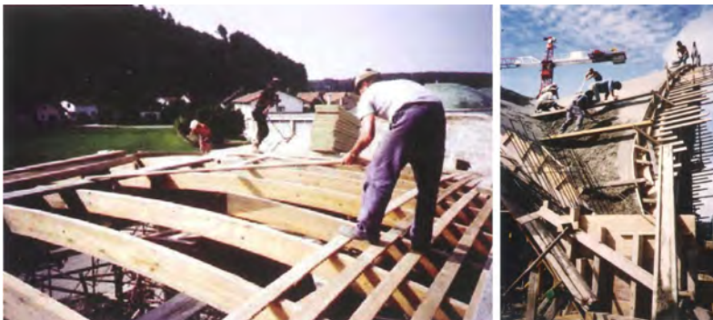
Figure 2.1: Timber formwork construction and casting of Isler shells (taken from Bösiger, 2011)
