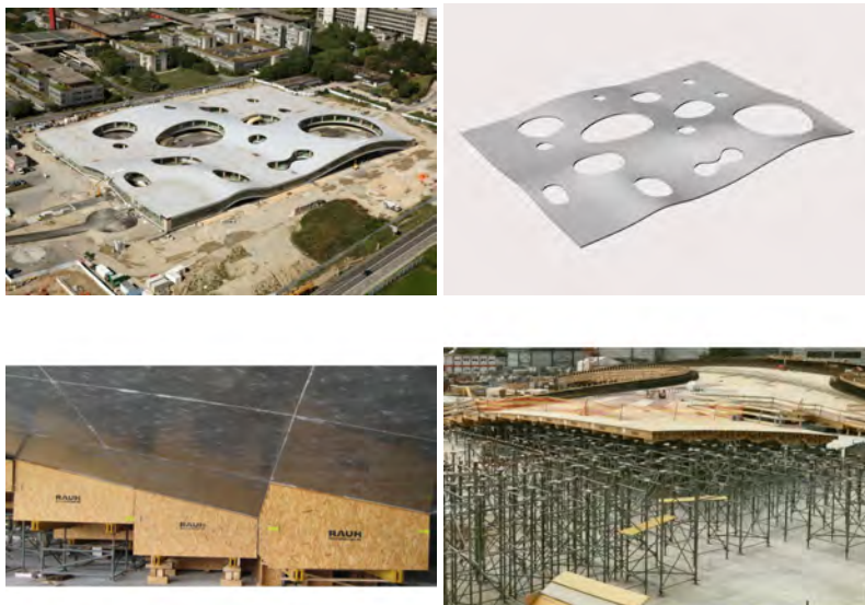
Figure 5.3: Rolex Learning Centre, EPFL, Lausanne - clockwise starting top left: the building as it was under construction around 2010; the curved CAD geometry of the concrete ground floor with a thickness of around 80 cm; the scaffolding system consisting of props and customized timber tables; a detail of the tables and the concrete surface after de-shuttering (images: wikipedia, RS, Weilandt et al., 2009, Dennis Cheung)
