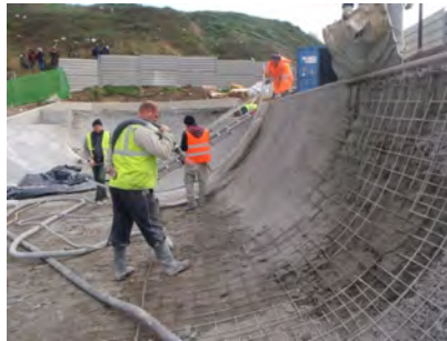
Figure 2.8: Spraying concrete on curved surface (confuzine.com)
