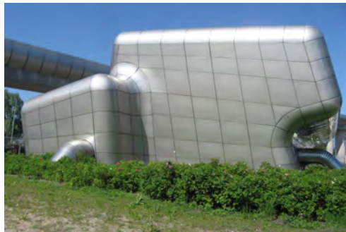
Figure 4.3: Explosion-formed stainless steel cladding, booster pump station Amsterdam, Group A architects, 2006 (image courtesy of flickr-jpmm)
