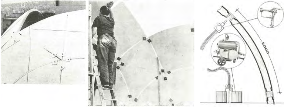
Figure 2.11: Two ways of connecting the triangular elements together, during assembly (left two images) and in the final stage (right) (Piano, 1969)
