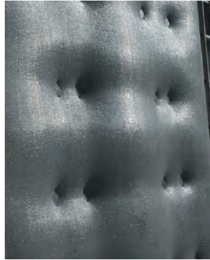
Figure 2.6: Concrete cast using fabric formwork (taken from Veenendaal et al., 2011)
