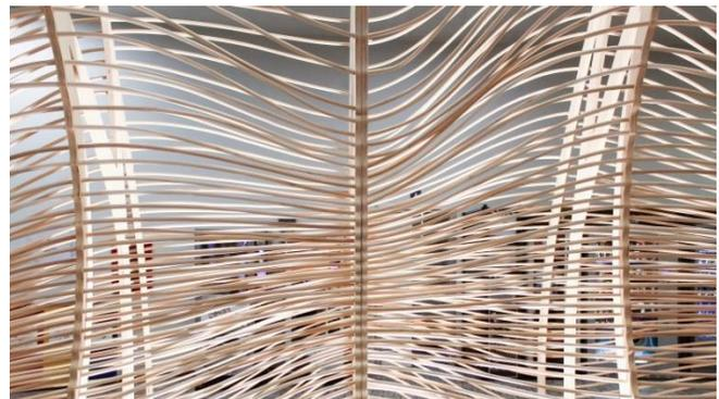
**Figure 19:** The variable density of rattan wefts generates a differential screening ratio along Weaving Enclosure surfaces
