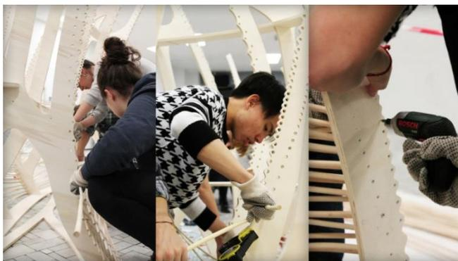
**Figure 17:** Manual work is still a fundamental step in the weaving process. Right. Screwing process for rattan post-tensioning
