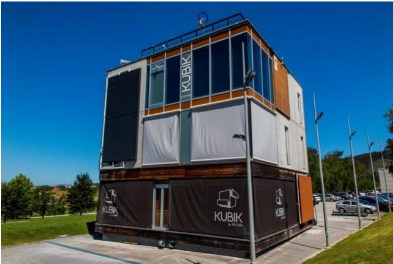
Figure 3: BASSE Sandwich steel envelope with at its pilot setup in the Kubik by Tecnia test facility [4].
