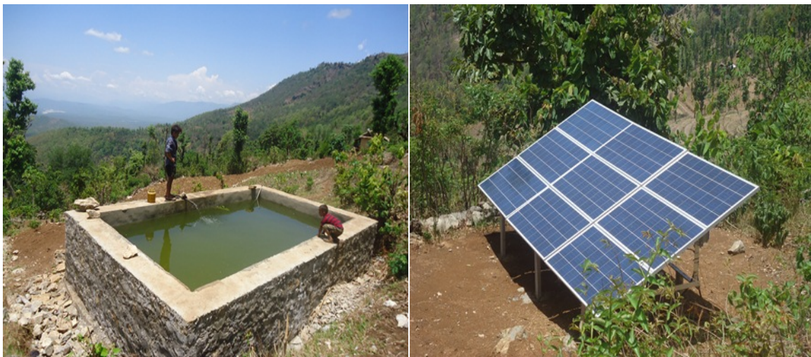
Figs. 11 & 12: PVWP system and water storage tank used for vegetable farming at Pokharikada, Surkhet, Nepal.
