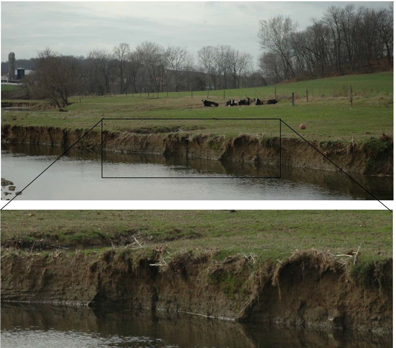
Figure 2. b) Eroding right bank along Big Beaver Run, Pequea Creek watershed, southern Lancaster County, ~100 ft upstream of a breached mill dam. Downstream flow is from right to left. All but several of the types of sediment production, storage, and transport can be seen at this location. Sediment might be moving down the hillslope during storms as slope wash, and the small channel on right bank (top left in bottom enlargement) could be considered as a rill. Bank erosion is extensive, and is associated with vertical fractures along which slabs of cohesive, fine-grained mill pond sediment collapse. At least three fractures are shown here in the laminated and cross-bedded sediment. Uppermost part of bank might have some hillslope sediment derived from upslope. Undercutting is occurring at the base of the bank, below the water, where a gravel layer lies upon bedrock. Little to no storage occurs in the channel, as it is bedrock. Just downstream, however, a large gravel bar exists. We note that most channel storage along this part of Big Beaver Run is coarse gravel, whereas most legacy sediment storage is sand, silt, and clay. No active floodplain exists, as the channel is incised and flow rarely tops the high banks.
