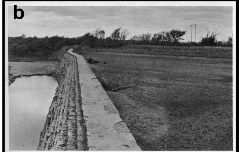
Figure 5. (a) View downstream of a USDA reservoir built in the 1920s (from Basile, 1971). (b) Same reservoir as in (a), after the reservoir filled with sediment in 1952 and was drained (from Basile, 1971). (c) An early 20th c. photo of Hammer Creek (see box of area in Figure 5d) shows a 10-ft mill dam and pond just upstream of an old mill building. The race is out of view, to the right. View is downstream, to the south. Today, the dam is breached and Hammer Creek has incised to the depth of the original valley floor. Remnants of the dam still remain. Hammer Creek was named for the continuous, round-the-clock pounding and hammering at the numerous forges and foundries along its length. (d) Historic (1864) map of part of Elizabeth township illustrates multiple dams and races along Hammer Creek. Photo in (c) was taken by Merritts of an original photo on the wall of the miller's house shown in the photo. Images in (a) and (b) are from Basile, 1971, and were flipped on the horizontal axis for comparison with (c). The map in (d) is from Bridgen's 1864 Atlas of Lancaster County, Elizabeth township.
