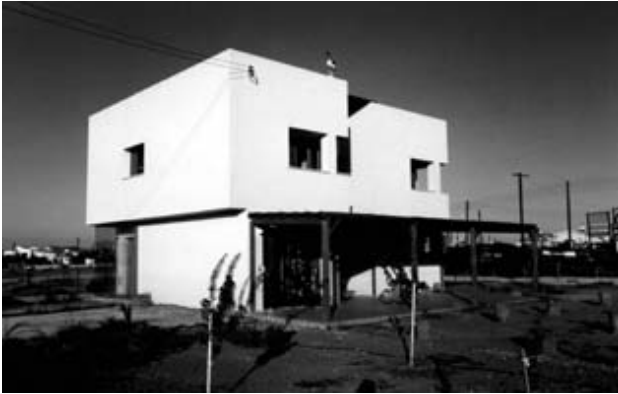
Photo 15. The twin pergola is used for both levels to protect from the southern summer sun. West and south facade
