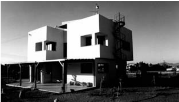
Photo 16. South and east facade
