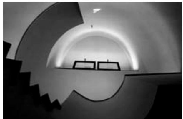
Photo 13. Staircase and clerestory window
