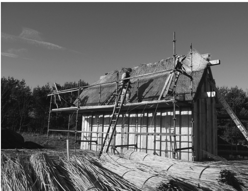
ILLUS. 45 Thatching, using a technique known as 'fleeking' in progress
