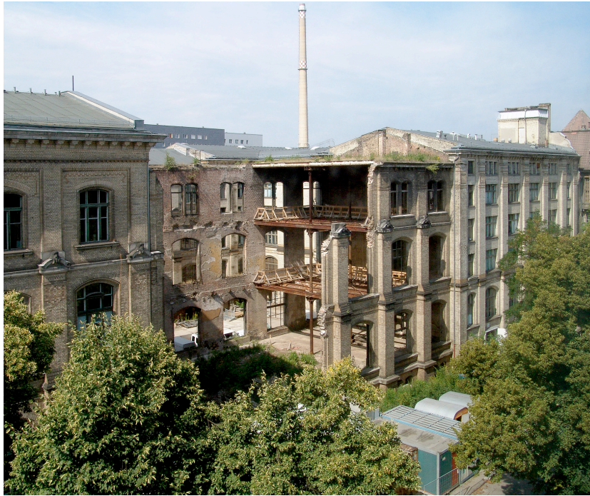
Figure 5. The ruined eastern wing in 2006. First preparations for the reconstruction
