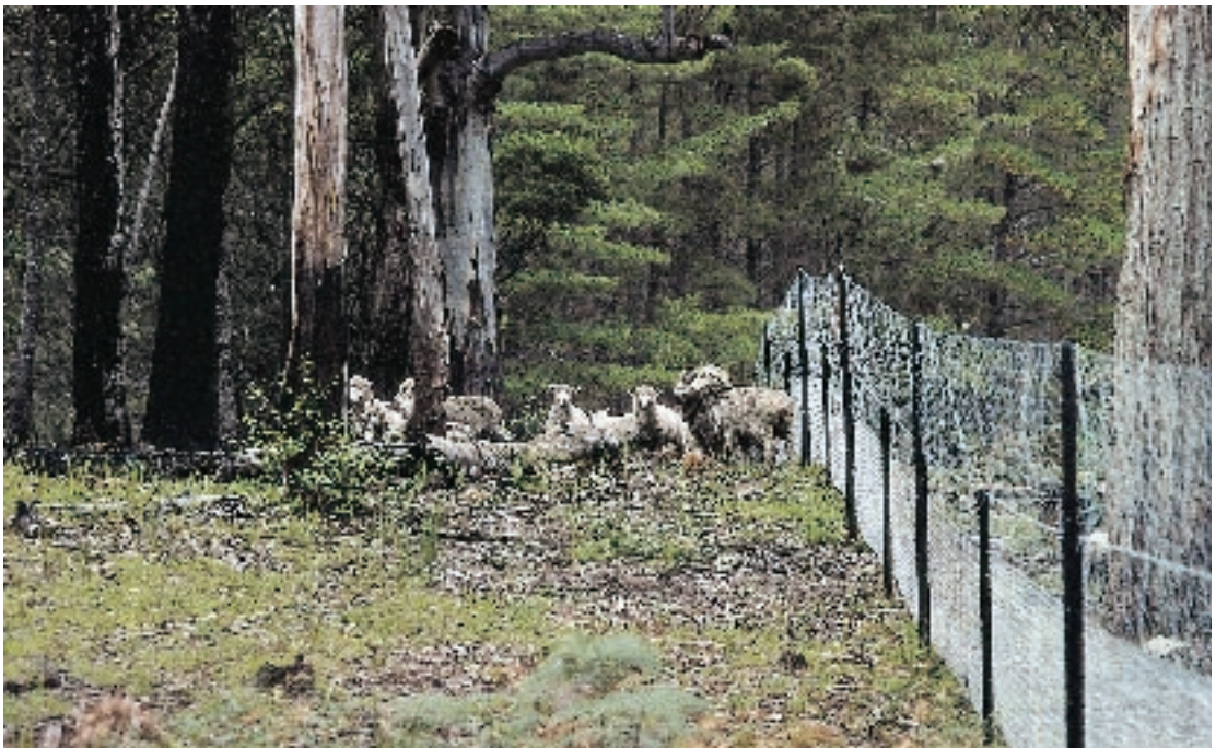
Figure 13: New wire-netting fences like this one are rarely constructed because of the cost. The fence is 1.8 metres high with the bottom half constructed with rabbit-proof netting and the top with lighter, marsupial-proof netting. A 25 centimetre flap of rabbit-proof netting is either buried or laid flat on the ground to prevent wild dogs, rabbits and macropods from digging under the fence (Source: P. Fleming).
