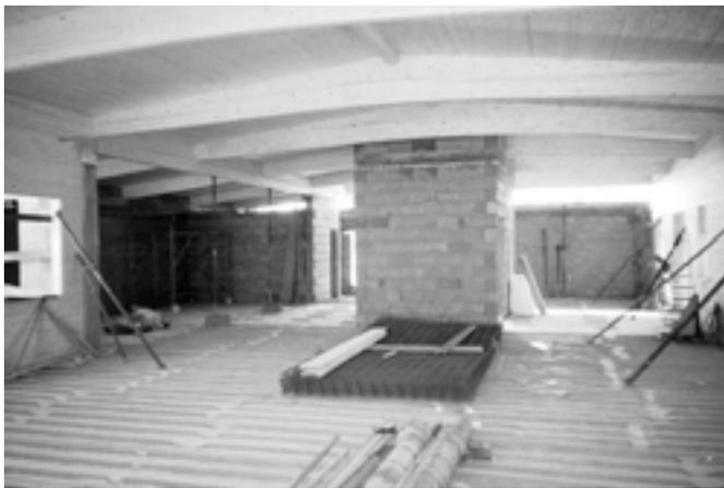
Figure 2. — Newly constructed commercial floor using a continuous steel mesh connector system.
