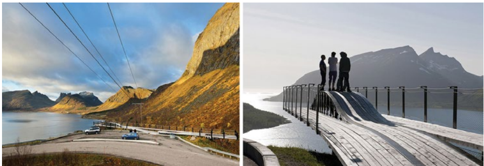
Fig.02a and Fig.02b Cantilevered viewing bridge at Bergsbotn, Senja by Code: Arkitektur.
