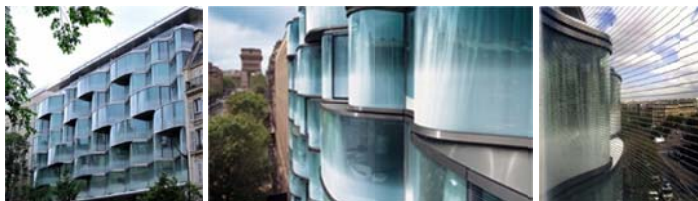
Fig.8: Arc de Triomphe hotel, the lines of fritted glass gradually change from bottom to top, (Kristal 2011)
