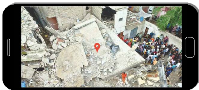
Fig. 5. Aerial View of a Collapsed building.
