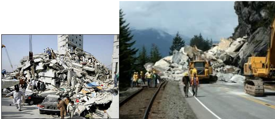
Figure 3.3 Destruction of infrastructure due to earthquake
