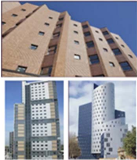
Figure-4. The applications of modular construction for high-rise and multi-story construction.
