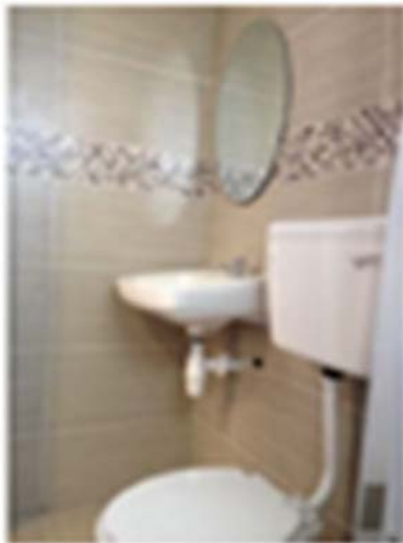
Figure-16. Finishing and fittings installation.
