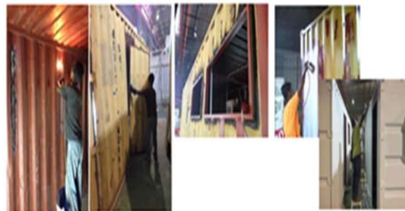
Figure-14. Cleaning, cutting and primer coating works.
