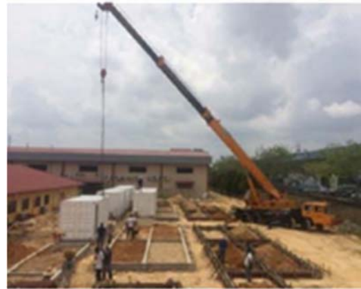
Figure-19. Site installation of the shipping containers at the site.
