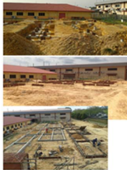
Figure-18. Earthwork and foundation preparation.
