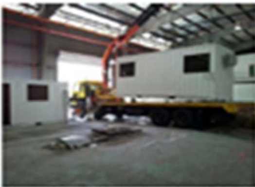
Figure-17. Transportation of the containers to site.
