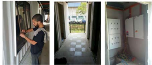
Figure-23. Mechanical and Electrical (M&E) and fittings installation.
