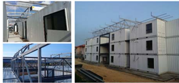
Figure-22. Site installation of roof structure and coverings.
