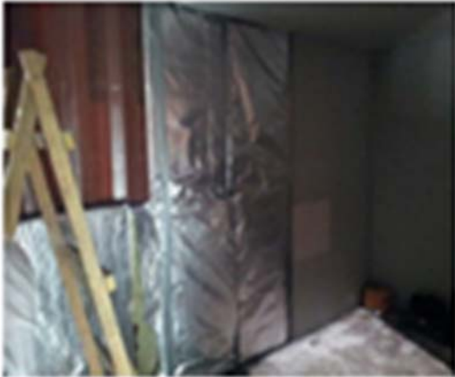
Figure-15. Insulation, electrical and piping installation.
