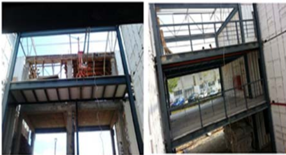
Figure-21. Site installation of floorboards and railings.
