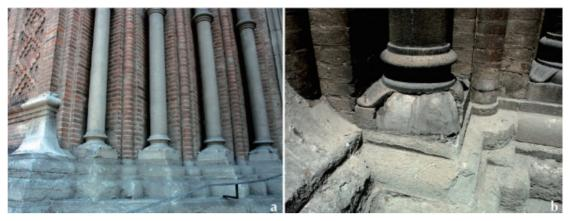
Figure 6. a) Precast concrete columns on a weak sandstone base in the Sacro Cuore Church in Bologna, Italy; b) detail of a column where the external cement-based mortar layer is detached from the concrete core
