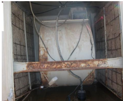
Figure (3): The affect of the cumulated salt on the evaporative cooler (inside the cooler)
