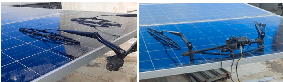
Fig. 5. Cleaning solar panels by car wipers, a pilot project.
