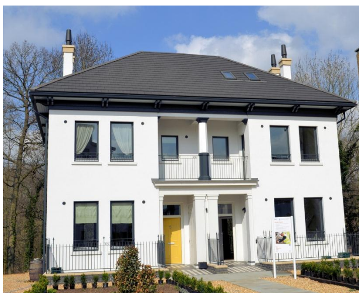
Figure 8: BRE Innovation Park, Watford, The Prince's House
