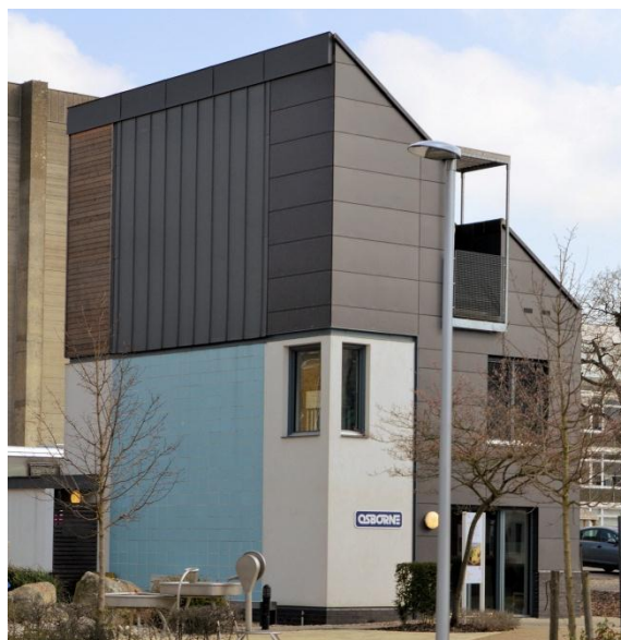
Figure 9: BRE Innovation Park, Watford, Osborne Affordable House
