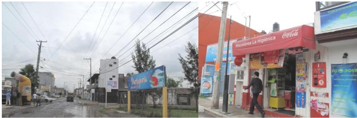
Image 14 Degradation of streets and transformation of social housing in the land reserve Quetzalcóatl, Source: author (2014)
