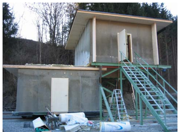
Figure 1: Test facility at KLH Massivholz GmbH with the ground floor moved out
